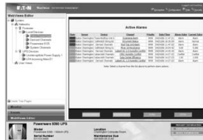
Device Monitoring — Alarms
